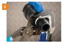
Using a pipe wrench or multigrips on the end caps only, further screw the ball valve until tight. Where necessary, ensure the thread is held stationary to avoid it from moving. Do not use pipe wrench or multigrips on the body of
