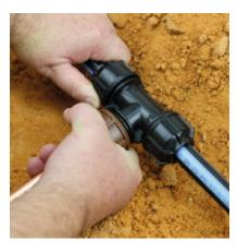
**6.** Tighten the nut by hand and finish using a wrench. Remember to check that the nut is tight against the body flange.
