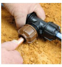
**5.** Insert the copper pipe and push past the rubber seal up to the mark indicated.
