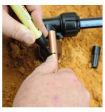
**4.** Cut copper pipe square. The fitting is preassembled and ready to use. Mark the depth of copper using pipe stop marking or body flange as a visual indicator.
