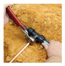
**7.** The nut should be tightened firmly with a wrench.
