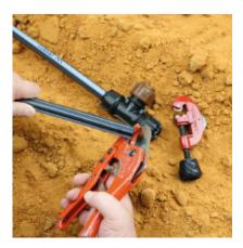
**1.** Cut pipe square. Ensure the pipe is free from sharp burrs. Chamfering or lubrication is not required.
