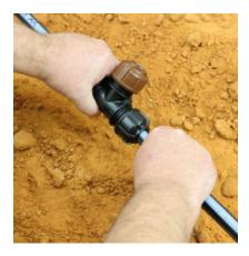
**3. Pipe Insertion**Insert the pipe and push it past the o-ring.
