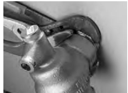
**3.** Using a pipe wrench or multigrips on the hex of the valve, screw it into the female thread until tight. Where necessary ensure the female thread is held stationary to avoid it from moving.
